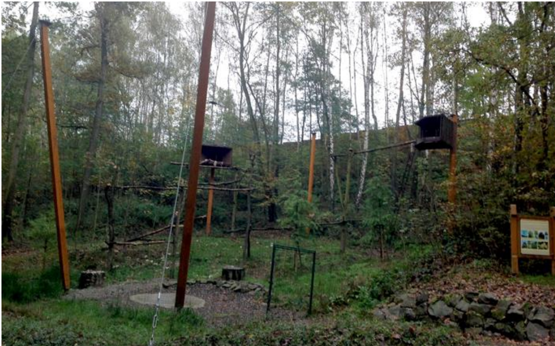
Picture 1: View from the entry. The huge Bearded Vulture facility has only wooden pillars for sustain the mesh.
