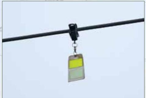
*Bird flight diverter structure designed in such a way so as to reflect light while rotating*
