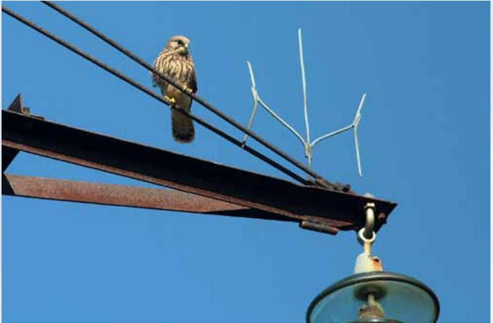
*Common Kestrel juvenile on electricity pylon with protective measures with Wishbone and Saucer type protection*
