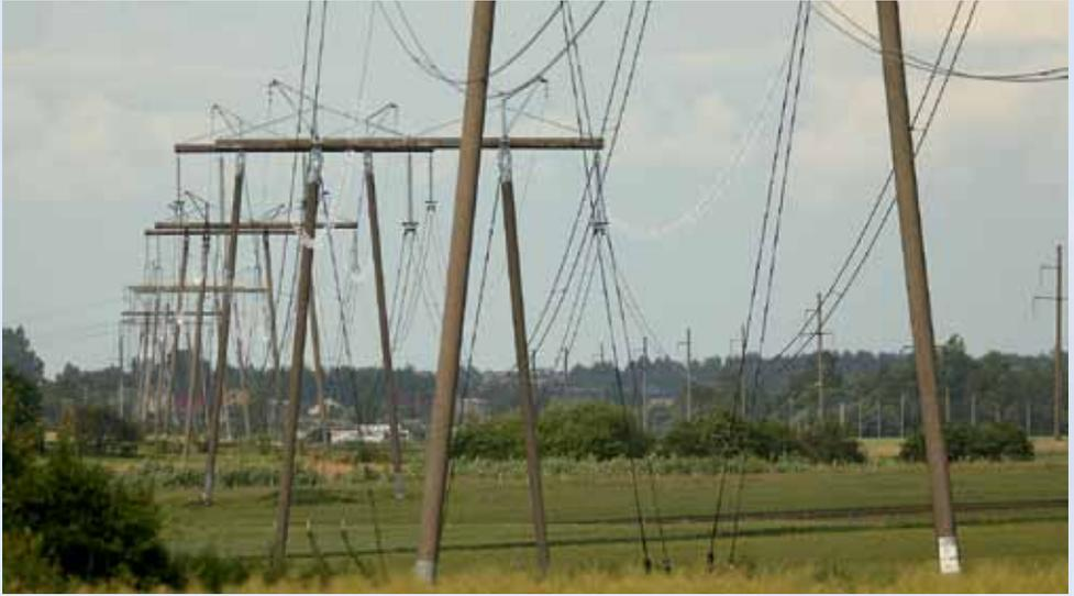
*Visibility of wires improved with the help of white coils*
