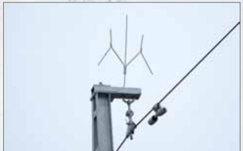
*The wishbone prevents birds from landing above the wires*
