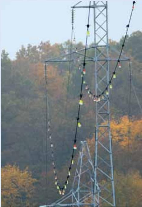
*The bird flight diverters improving visibility of high-voltage electricity transmission lines in Kaunas near hydroelectric power station*
